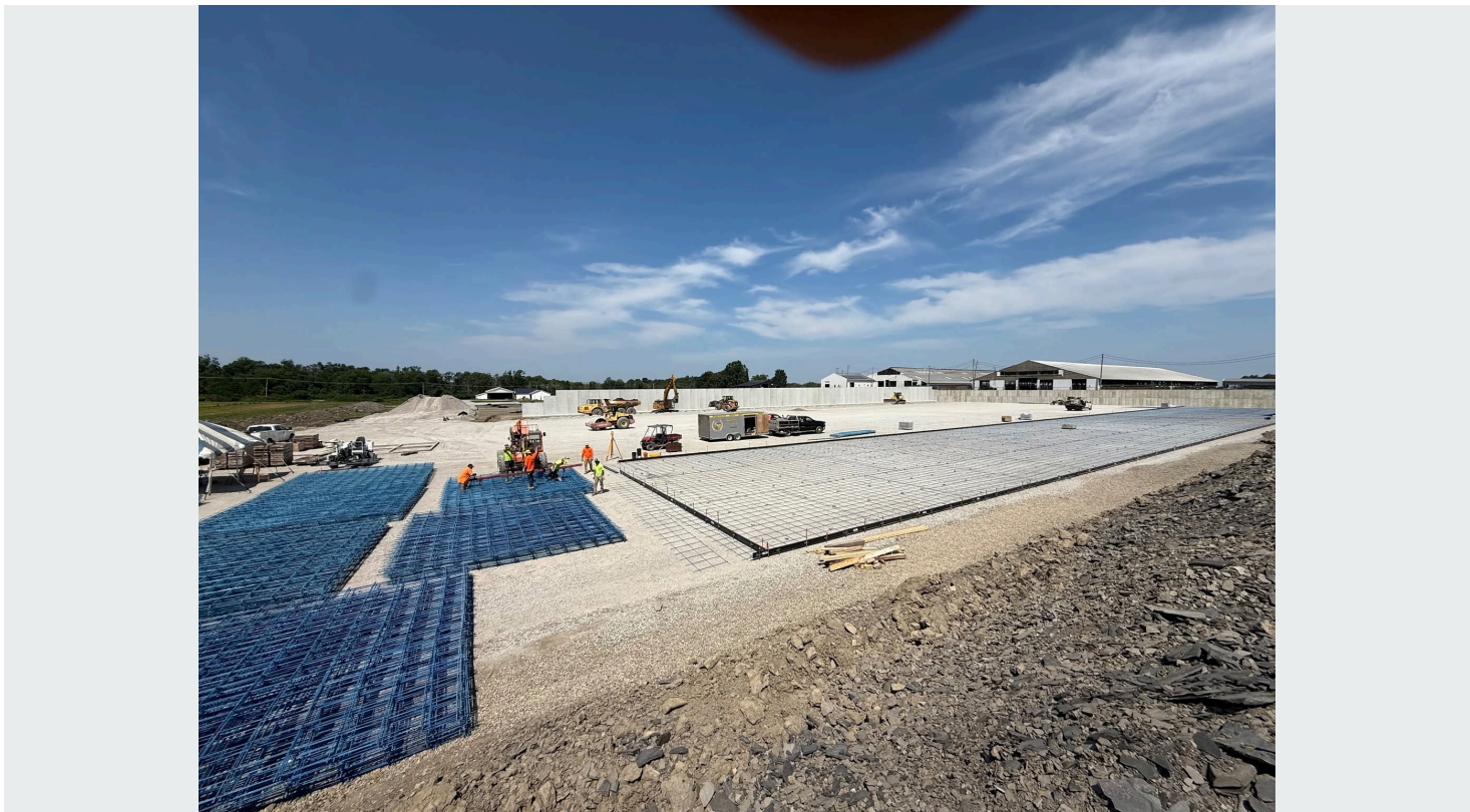
LARGE-SCALE REINFORCED SLAB PREPARATION / ACTIVE PROJECT PHOTOGRAPHY
