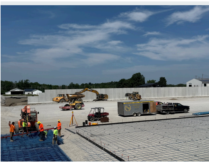
LARGE-SCALE CONCRETE OPERATIONS
