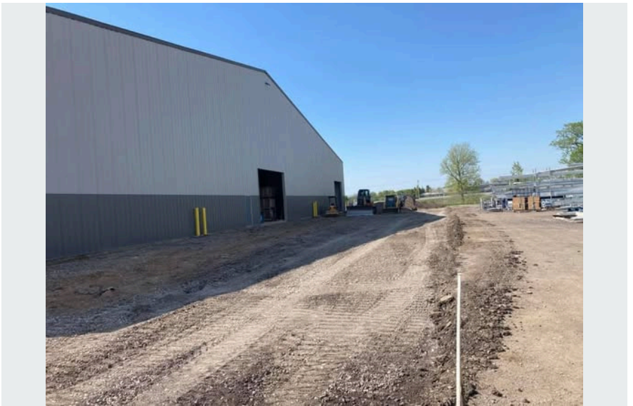
EXTERIOR CONCRETE FINISHING
